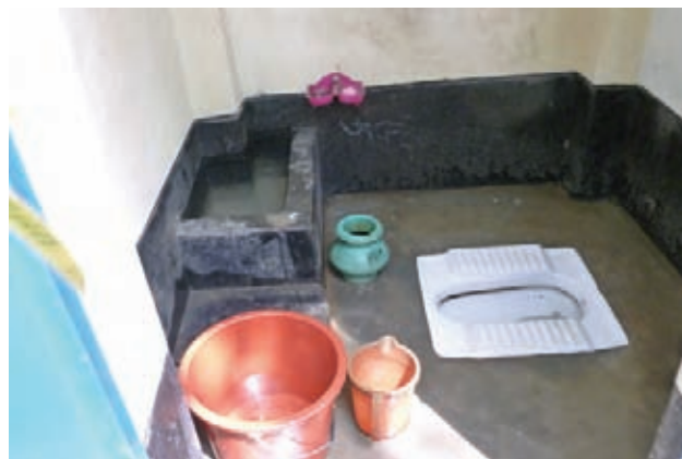
Figure 8 Additional space in school latrine cubicle for washing and drying sanitary napkins in Sylhet, Bangladesh A George 2012
